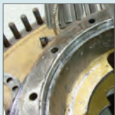
Pitting on bearing
