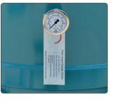
CJC<sup>™</sup> Filter Insert Change Sticker The sticker is placed next to the pressure gauge. Follow the guide, how to place the sticker.
